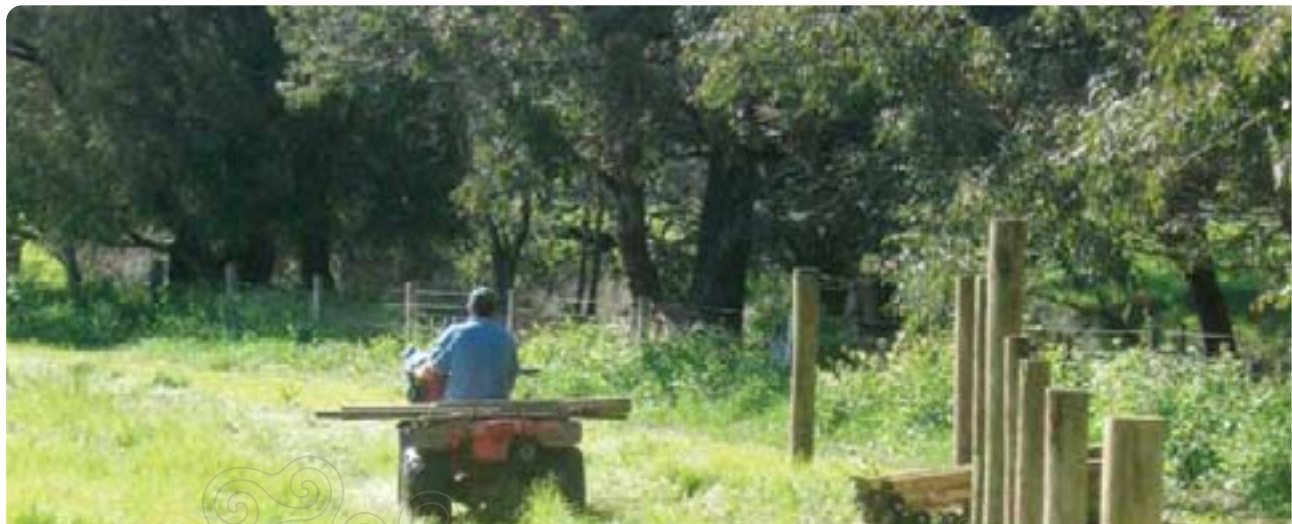
Commencement of re-fencing works to protect the river.
