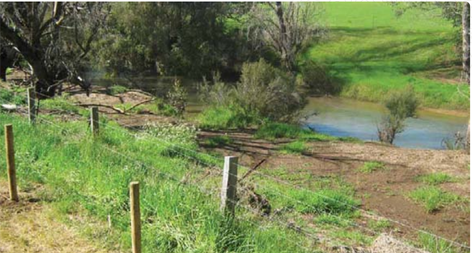
Following re-fencing, weed control and planting was completed through the Autumn and Winter of 2011.
